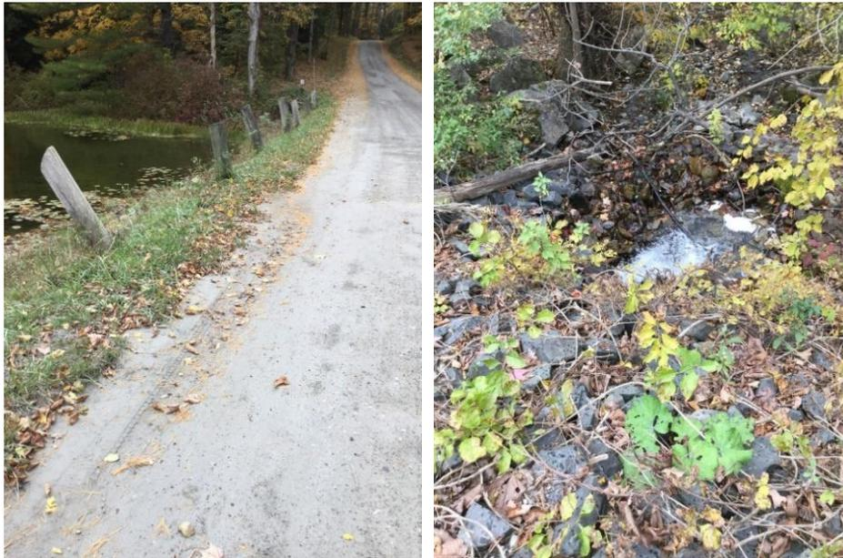
Figure 9. Culvert crossing on Rossiter Road which experiences flooding during heavy rain events. The inlet (left) grating is partially covered by debris and the outlet (right) headwall may need further study.
