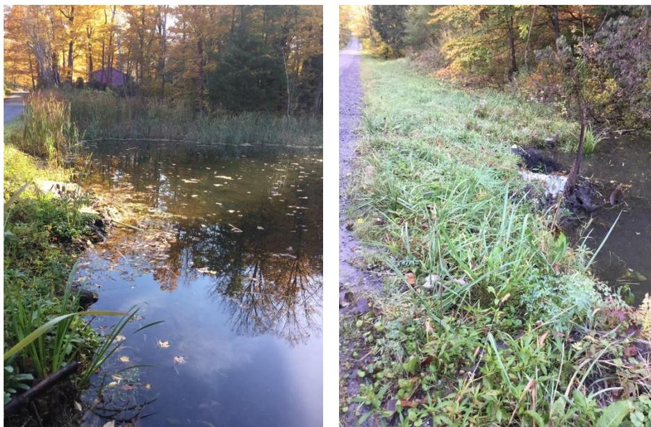
*Figure 10. Road-stream crossing culverts clogs by beavers along West Alford Road. WS.PA-8 (left) has an impoundment behind it. WS.PA-9 (right) has a small impoundment between it and a large beaver dam.*
