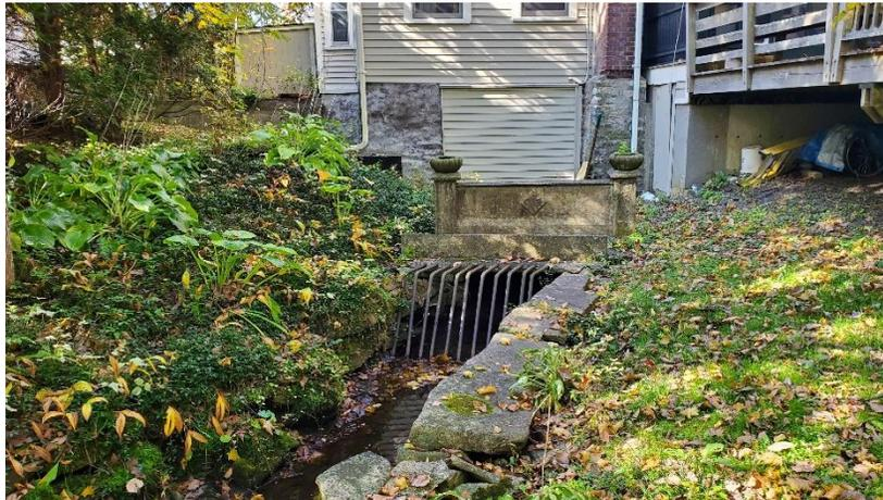
*Figure 8. The inlet to the culvert beneath a home in downtown West Stockbridge*
