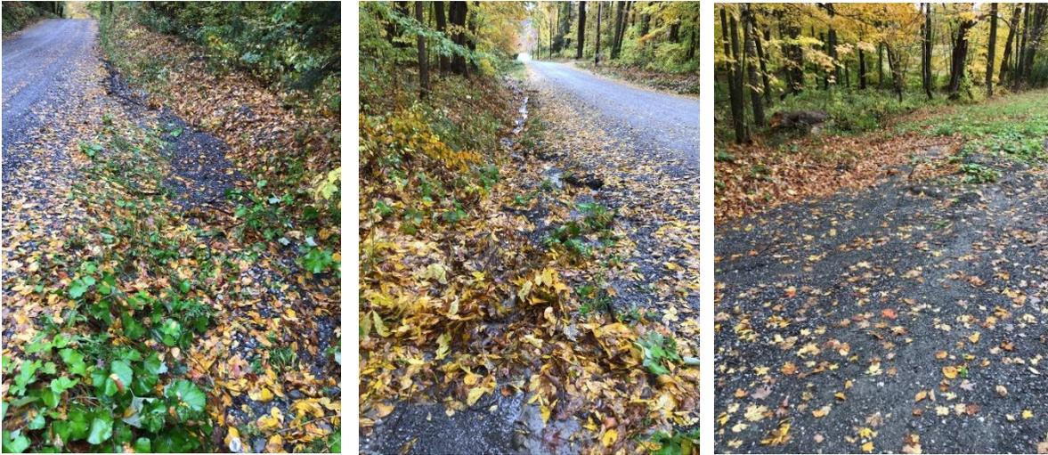
*Figure 3. Condition of the roads post-rain event on October 14, 2022. There is channeling on the north and south swales, looking downhill, of Red Rock Road (right and center). Accelerated flow down steep parts of Austerlitz Road bleed into the woods at the bottom of the hill, eroding the road (left).*
