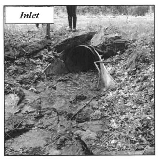
Inlet Shape/Type: Round Culvert/Wingwalls
