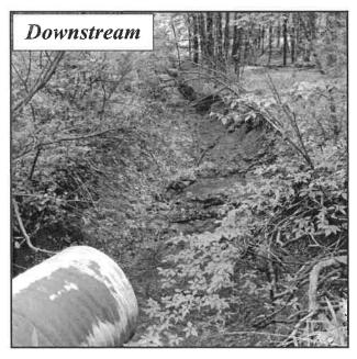
Crossing Comments: Severe erosion downstream; road sediment filling channel at inlet
