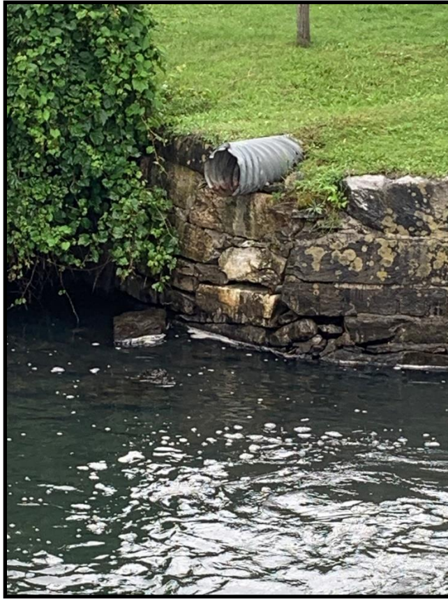
24. Area of deficiency: Undermined stone at base of right downstream masonry wall
