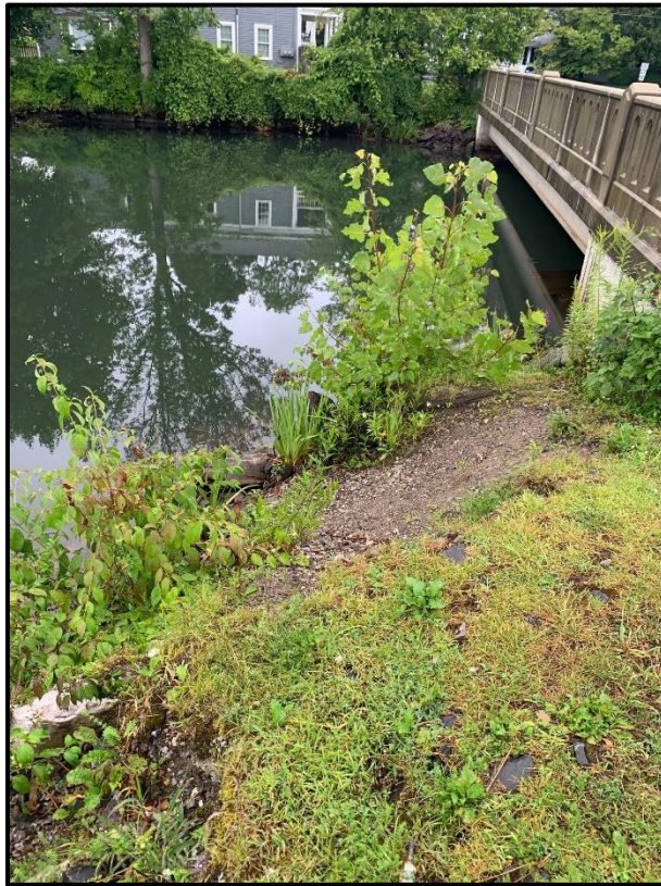
22. Area of deficiency: Erosion at right embankment at bridge end from upstream
