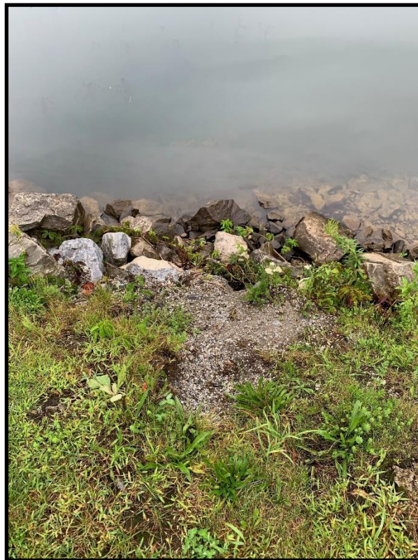
22. Area of deficiency: Erosion at right embankment at bridge end from upstream
