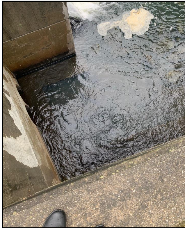
26. Area of deficiency: Boiling at base of hydro area
