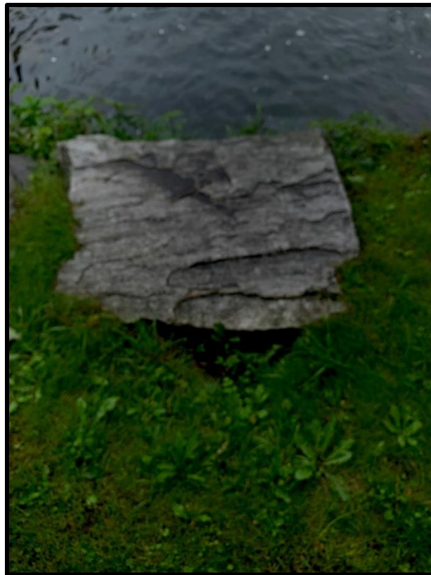
25. Area of deficiency: Sinkhole at right side of downstream masonry wall capstone
