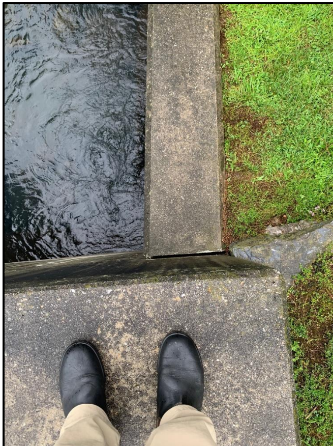
27. Area of deficiency: Deteriorated joint caulk at downstream concrete joint
